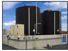
Thermoplastic tanks are manufactured using the latest butt welding technology and are fully compliant with standards such as BS EN12573, DVS205 etc depending on the customers specification.
