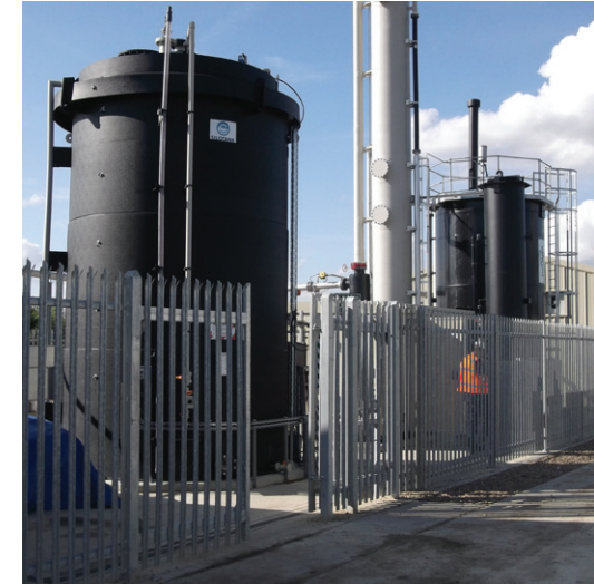
35,000 Litre Polypropylene Minitank, PP tank c/w PP bund - PAS Grantham McCain Foods, Lincolnshire, England. Tank is storing 33% Sodium Hydroxide.
